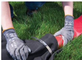
Included hose clamp is threaded through precut openings.
